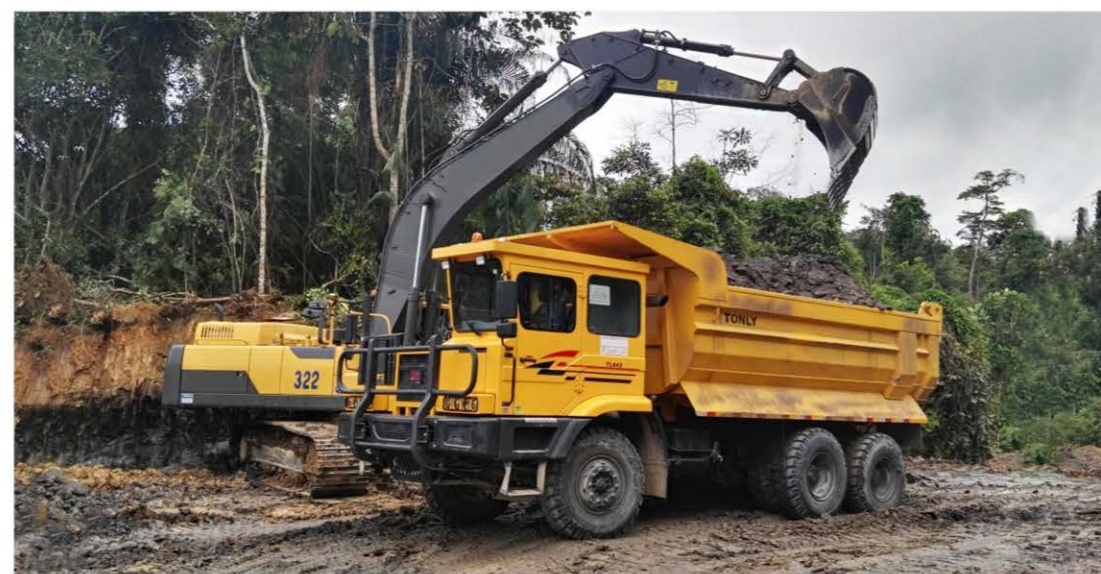
Malaysia Coal Mine
